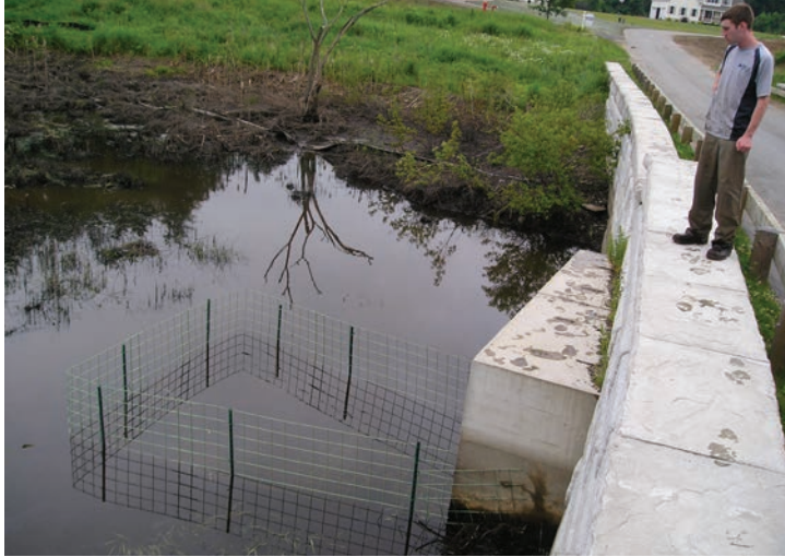
Trapezoidal protection fence in Westford, MA prevents beaver from blocking the culvert. (Photo: Mike Callahan/Beaver Solutions, LLC)
