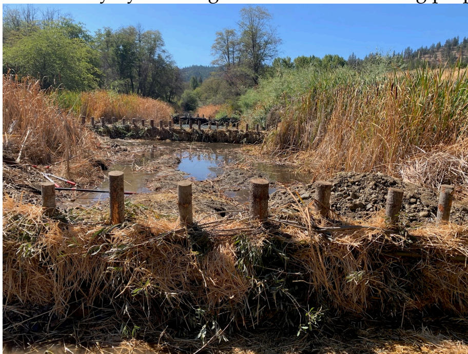
Fig. 4.4 3 of the 4 BDA's working in series on Sugar Creek. Each BDA took about 2-3 hours with 15 people
