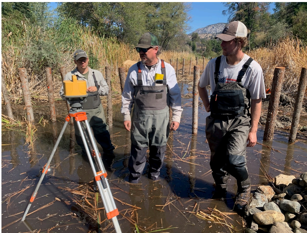
Fig. 4.6 Nick learning how to use the laser level to ensure the BDA is the same height all the way across
