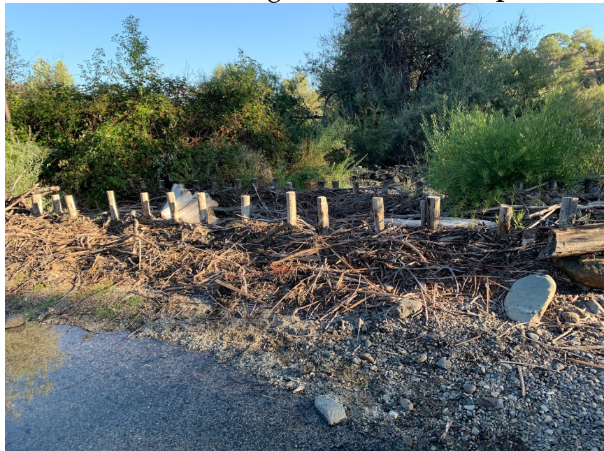
Fig. 4.5 The first ever BDA built in California at Sugar Creek and behind it a couple smaller supporting BDA's
