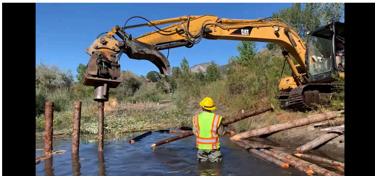
Fig. 4.2 The excavator pounding posts with a vibratory plate attachment
