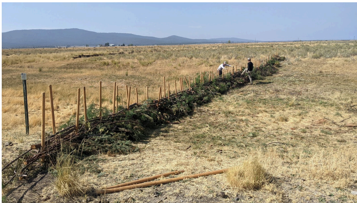
Fig. 3.6 Cooper and Nick working on the longest BDA built at Mc Arthur measuring in at 90 feet
