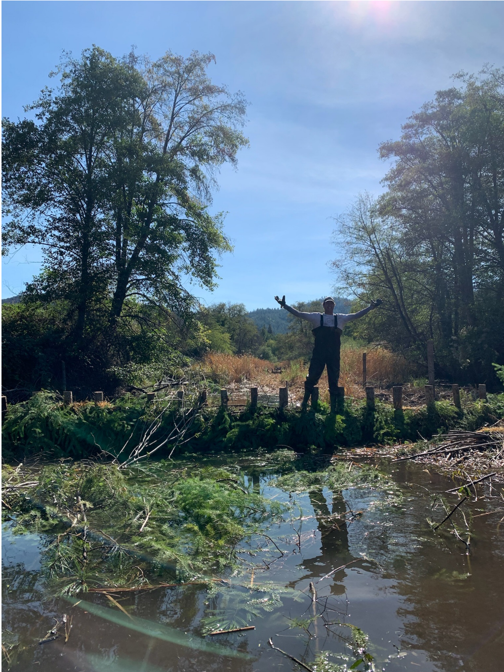
Fig. 2.1 Cooper stands atop a newly constructed BDA in the Scott River, Etna, CA
